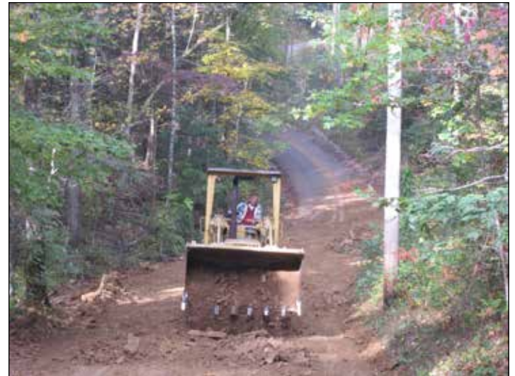
Tom makes road repairs on Walnut Flats Road.
